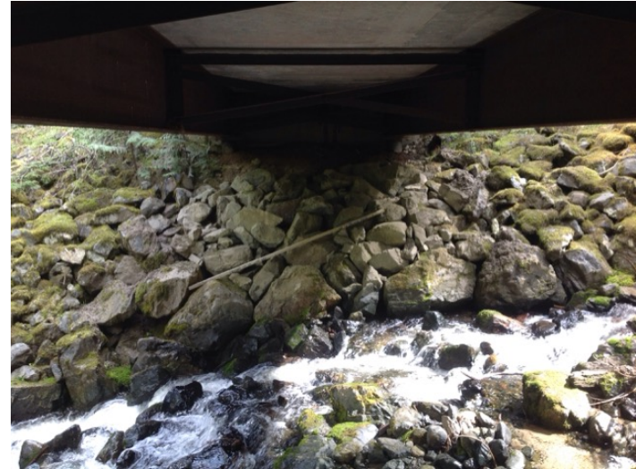
Right Bank Abutment when facing downstream
