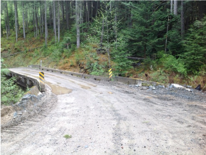
Approach from Left Bank when facing downstream
