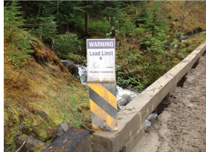
Load rating sign
