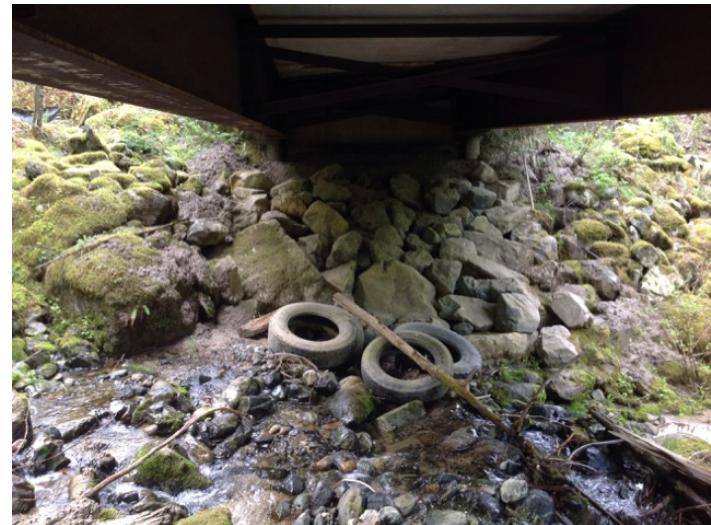
Left Bank Abutment when facing downstream
